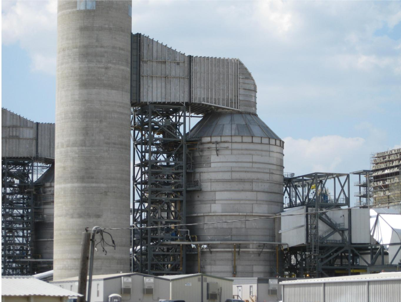
**Scrubber remove SO<sub>2</sub> from flue gas**
